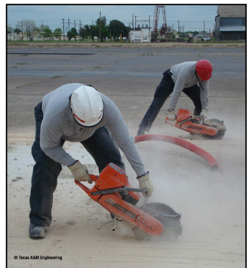
Figure 1. SMEs cut airport runway concrete using multipurpose cutoff saws and test blades.
