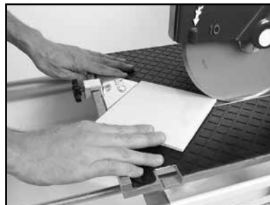
(E) Perform the cut. Turn the motor OFF when work is complete.
