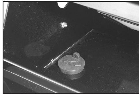
Fig. 21 Inspect Drain Plug
