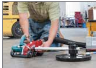
Attach saw to pivot bar
