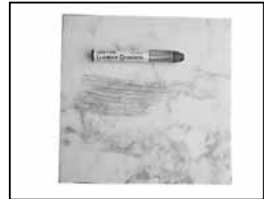
(F) Dry surface then rub the surface with a lumber crayon to deter- mine the depth of the remaining scratches.
