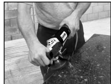
(I) Repeat Steps A through F using fine grit discs to complete polish- ing of the surface.
