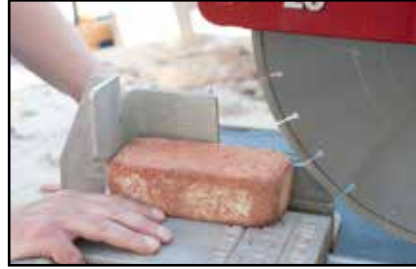
Place brick on riser and start saw.
