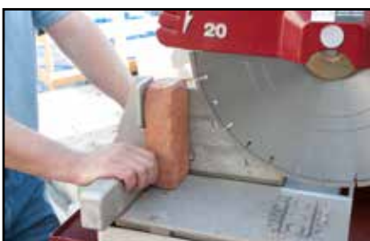
Pull table back through brick and flip brick vertically.
